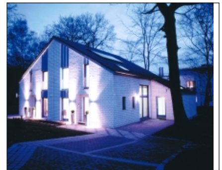
The inHaus complex integrates all of the functions of an experimental, networked dwelling house and a workshop of the future. Practically all of the installations are hidden behind the walls and tiles © Fraunhofer IMS / Axel Struwe.
